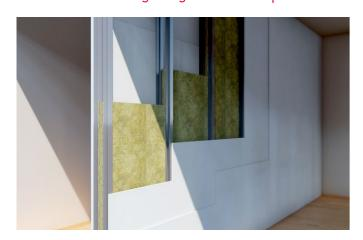
Studs: 70mm metal 'C 'studs at 600mm Centres
