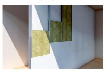
Studs: 70mm metal 'C 'studs at 600mm Centres
